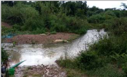
N218.9m unaccounted for on this poorly executed project nominated by Sen. Agboola for Oyo state.
